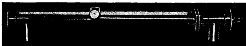
FIG. 12-37.—Side-outlet \frac{1}{2} -in. variable attenuator.
